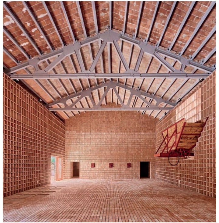
Arqitectura Camps Felip: Renovation of the Flix Agricultural Cooperative, Tarragona, 2023. Photo: José Hevia
